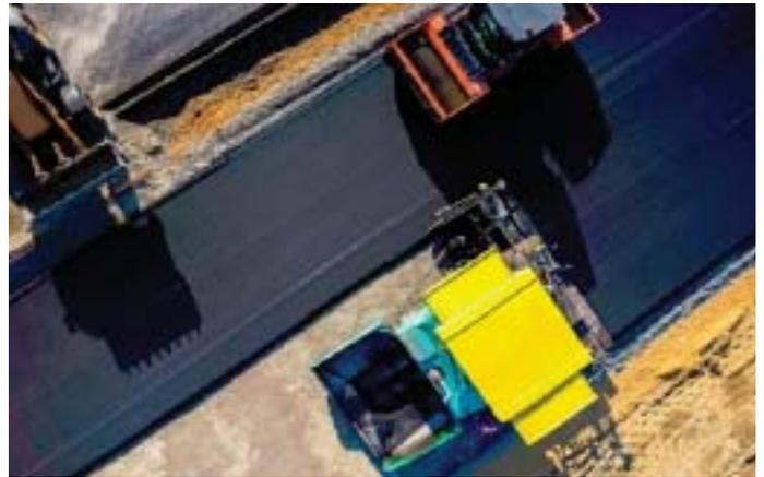
Bitumen or asphalt is a black semi-solid viscous material traditionally used in waterproofing or as a mastic or glue, but now is principally used in road pavement construction. The global bitumen industry provides 85% of all bitumen mixed with aggregate filler for use in asphalt pavements. Only 10% is provided for roofing, waterproofing and sealing [1].
